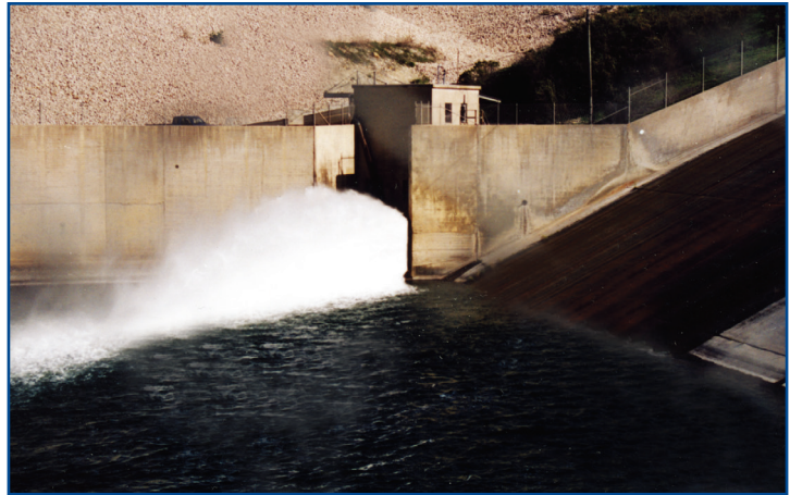
Free discharging fixed cone valve
