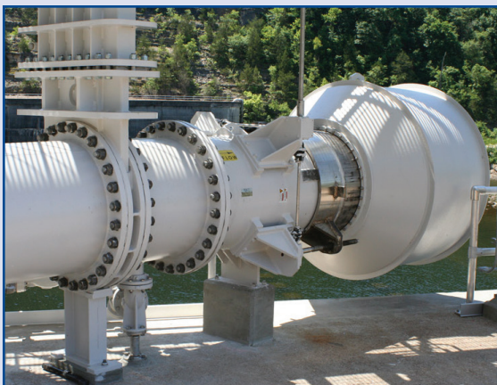
30" Fixed Cone Valve with Hood
