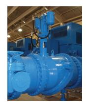
offering to those customers who require specialty valves for applications where opening and closing times are critical to control flow reversal and reduce water hammer.
